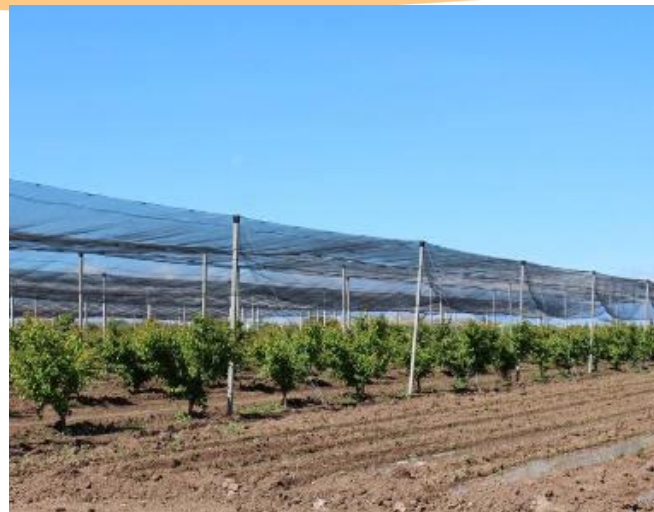
Installation of anti-hail nets
